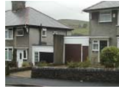
Gaps in the street frontage will allow views into the open countryside beyond
