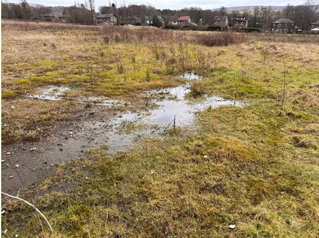
Photo 3: Surface waterlogging on the west of the site at time of the visit (February 26).
