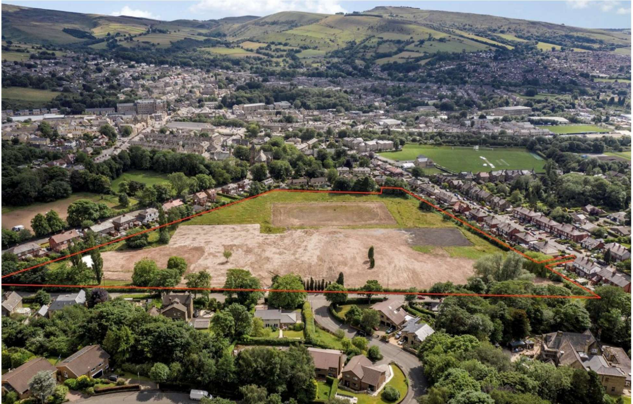
Figure C: Drone photograph courtesy of Derbyshire County Council of former Glossopdale Community College site post demolition (view south) shows much of the area is covered with demolition rubble.
