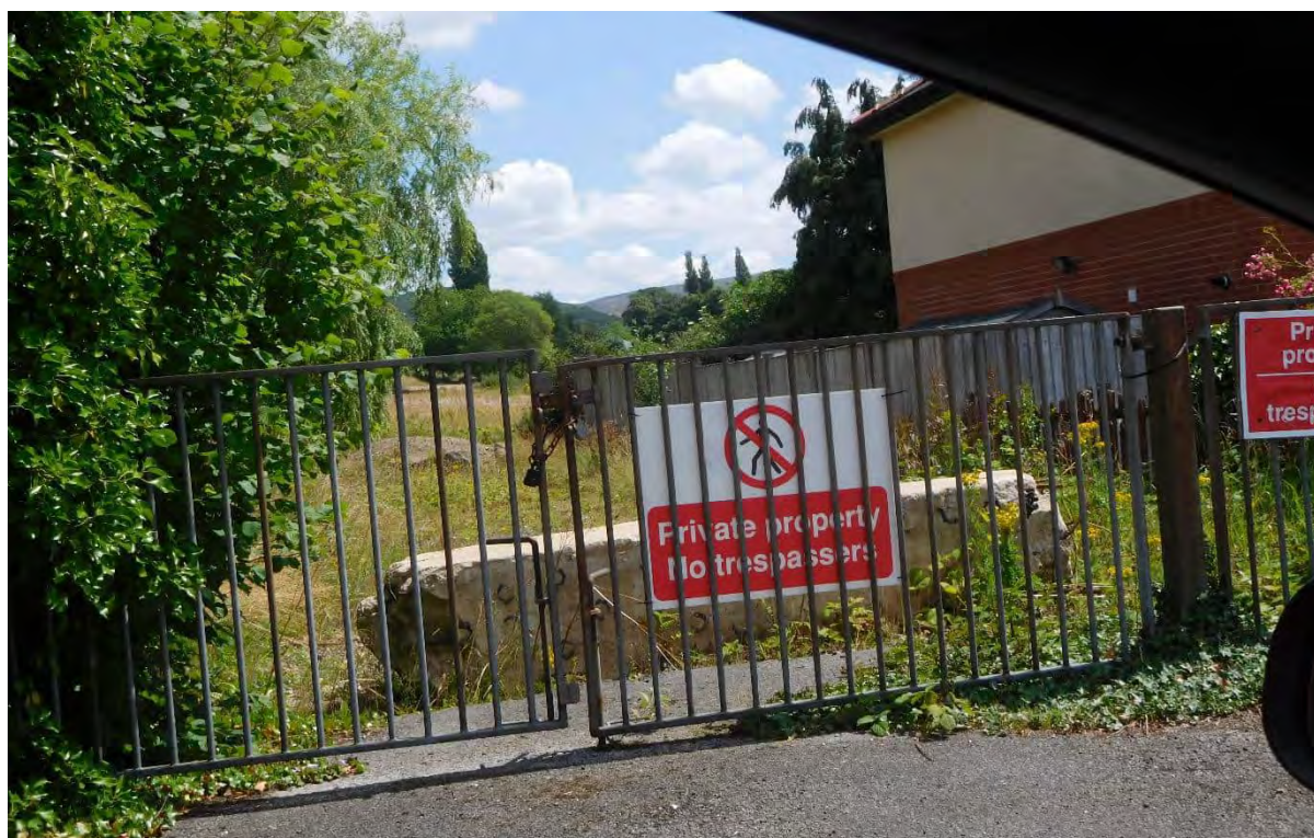
Figure C: Existing Access Point off North Road
