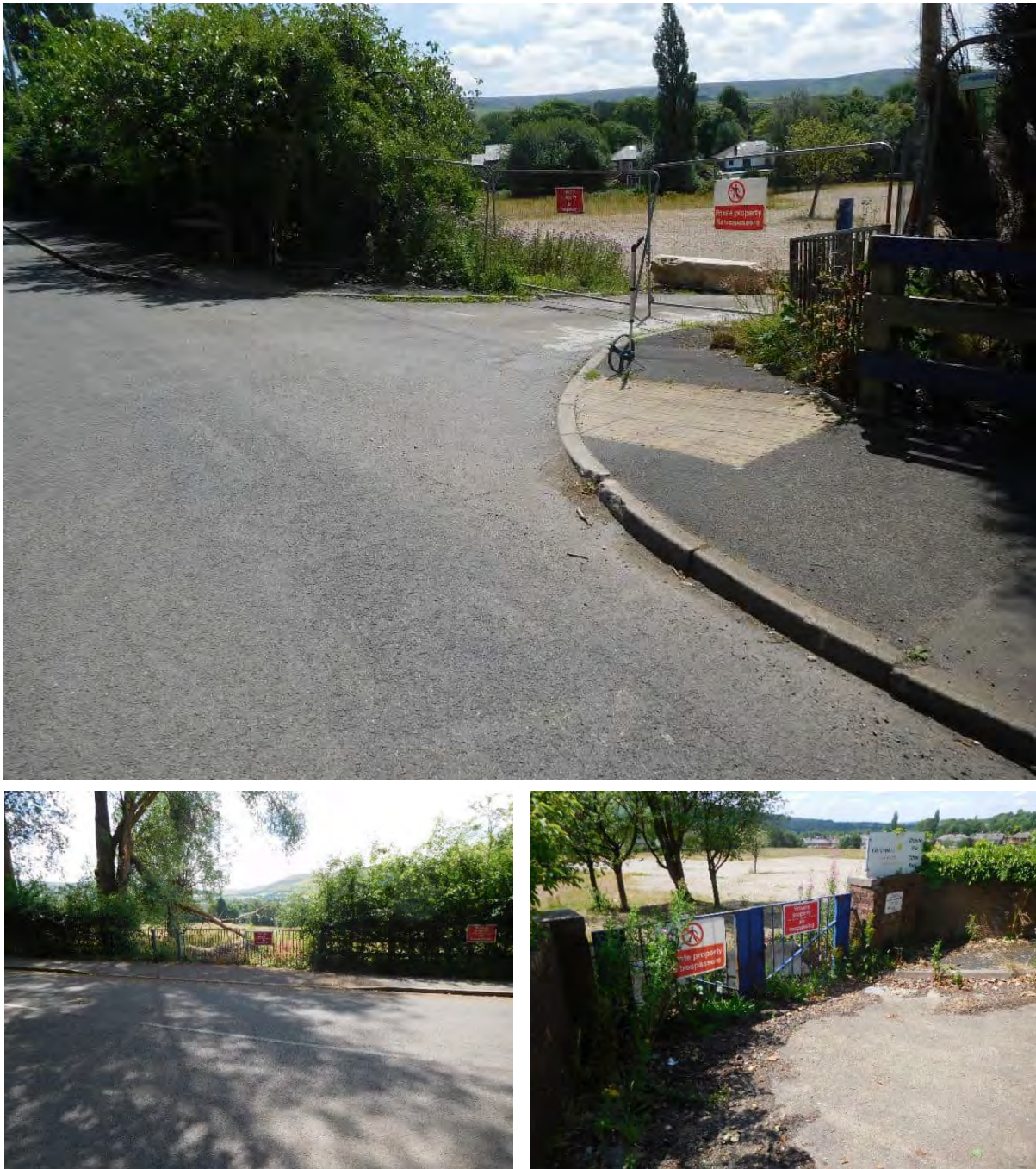
Figure B: Existing Site Vehicular Accesses from Talbot Road
