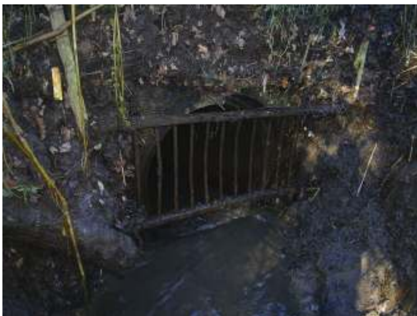
Inlet to 900mm Culvert
