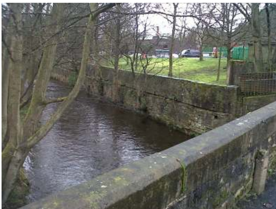
View of Birch Vale PEZ from Bridge over River Sett
