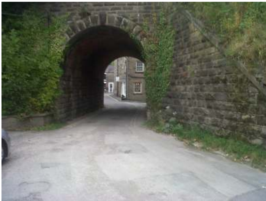
Wharf Road railway bridge
