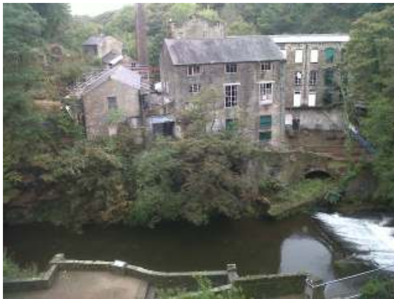
Fig 4.10.1: Torr Vale Mill with upstream weir
