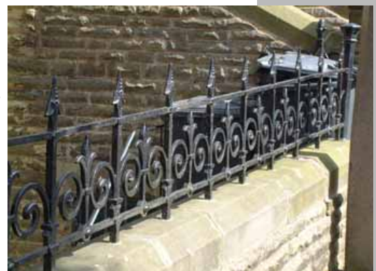
▲ Wrought iron railings
