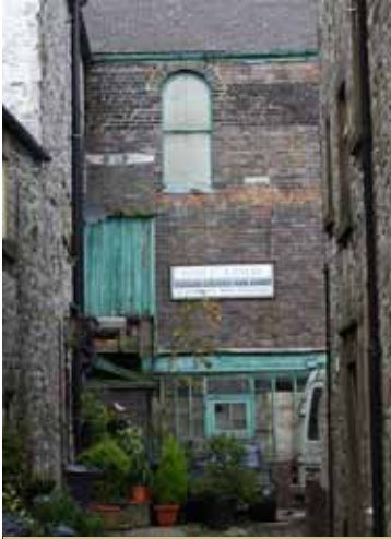
▲ Workshops at the rear of Torr Street
