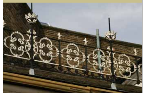
▼ Cast iron balustrade
