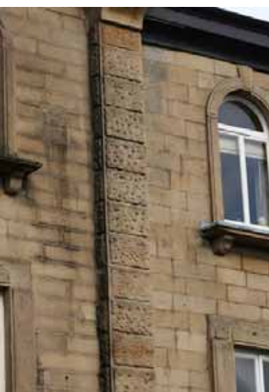
▲ Punched quoins / pilasters at The Quadrant
