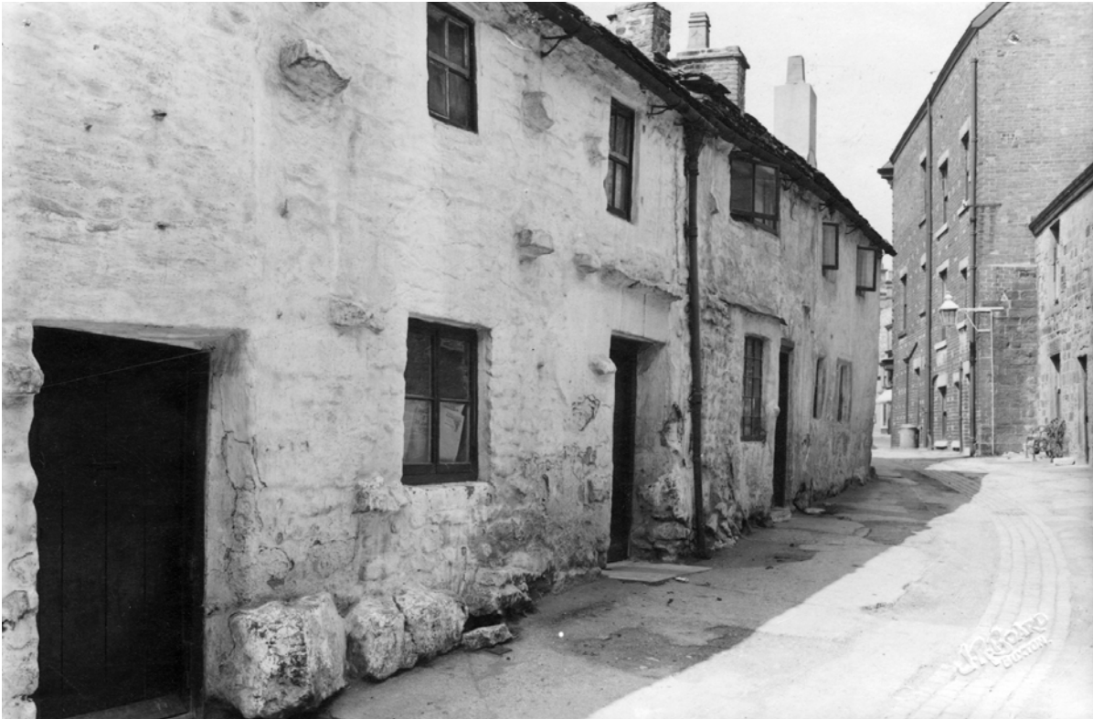
▲ Pl. 3 - Church Street - 19th century view of rubble limestone cottages, painted with traditional limewash (BMAG)
