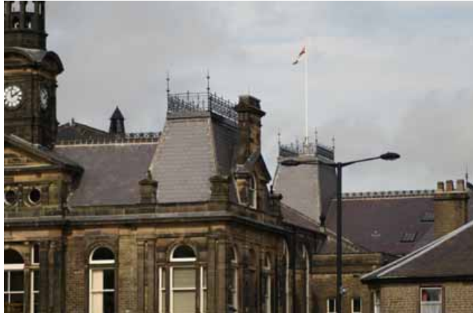
▲ Roofscape of the Town Hall - pavilion mansard roofs enliven the skyline and create depth
