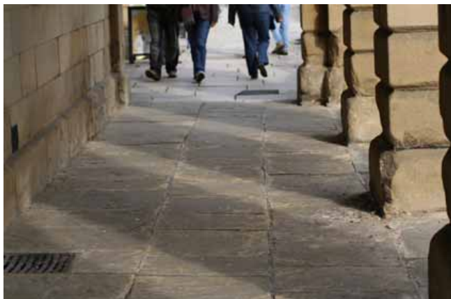
▲ Paving flags under the arcade - The Crescent
