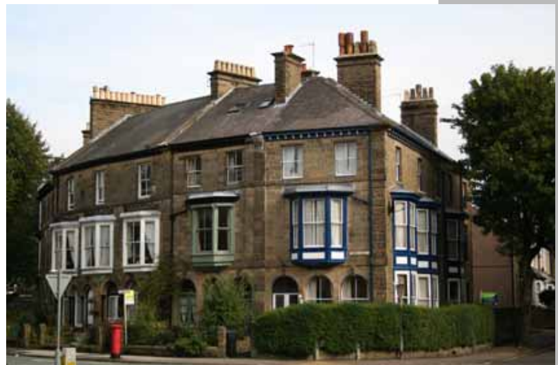
▲ Nos. 1-5 Bath Road, incorporating cast iron columns and arched ground floor windows
