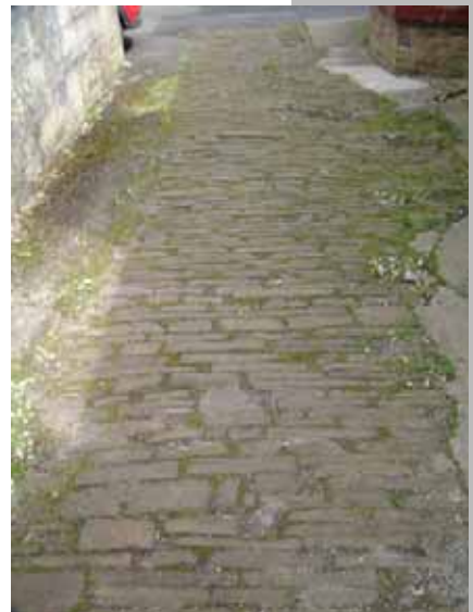
▲ Narrow gritstone setts - in front of the Old Wheatsheaf, Church Street
