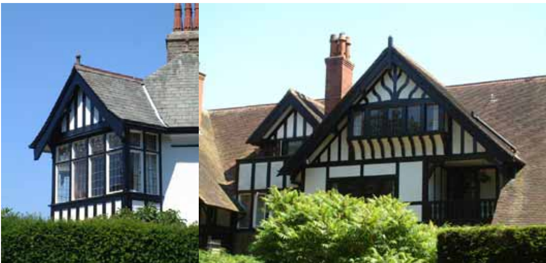
▲► Timber-frame concentrated on the gable-ends - Arts & Crafts houses
