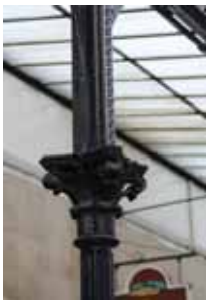
▲ Cast iron column
