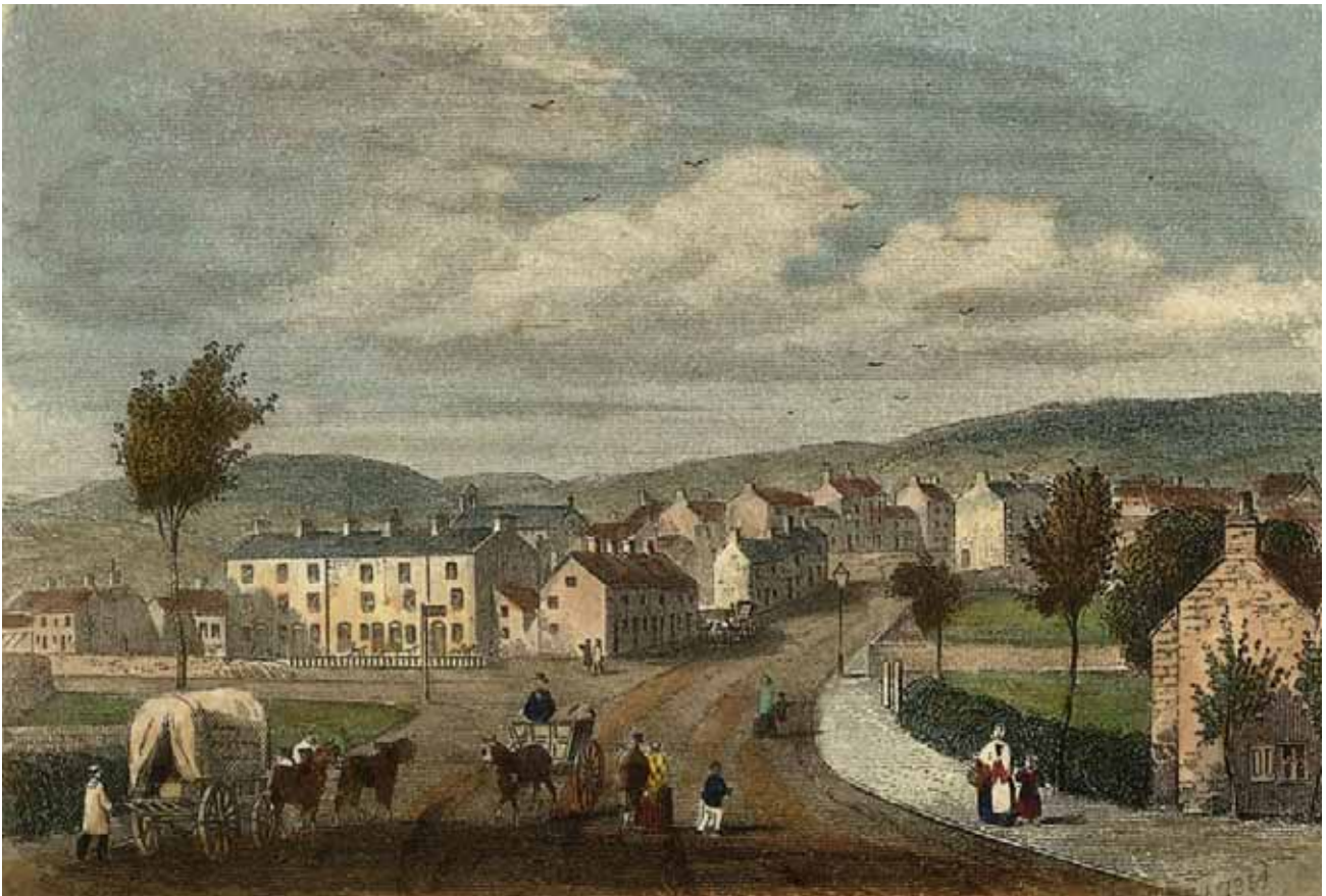
Pl. 21 - 1854 engraving of London Road and the bottom of High Street. The buildings following High Street are mainly two-storey. The main landmark is the three-storey terrace on West Road
