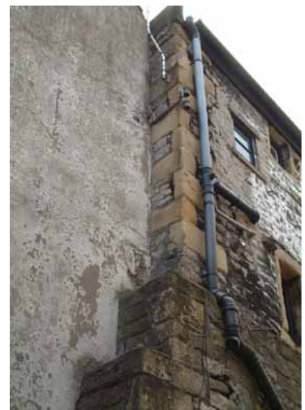
Rear of 14 High Street - stonework of an earlier phase is evident behind the main building
