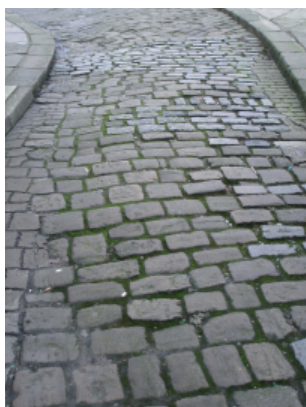
Picture 6 gritstone setts laid on Terrace Road
