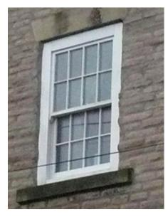
Figure 47 Eight-Over-Eight Sash Window, After c1850
