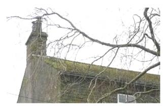
Figure 57 Stone Slate Roof With Stone Chimney and Clay Pots
