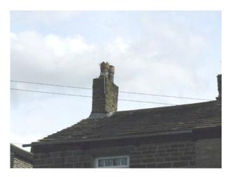
Figure 61 Stone Slate Roof With Stone Chimney and Clay Pots
