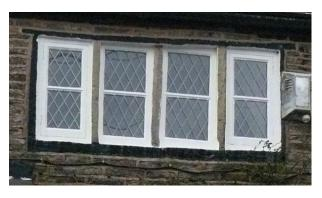
Figure 46 Side-opening Casement Window
