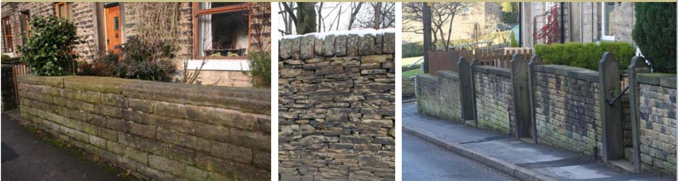
A few properties had a formal frontage, with a low, finely-tooled ashlar wall finished with decorative railings. An example of an ashlar wall, without its railings, survives at The Old Bank House. In some cases railings were also added to a higher coursed stone wall, where the ground was retained, such as at Nos. 101-103 Kinder Road, currently outside the conservation area.
