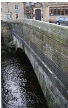
**Hayfield Bridge**, crossing the River Sett, is a fine bridge of 1837, designed by the Sheffield architect Samuel Worth. The single-span structure has distinctive horizontal bands of quasi-rusticated masonry.
