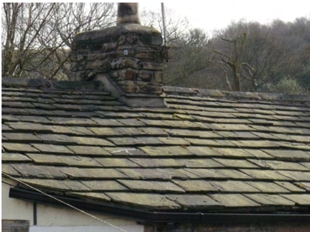
Figure 48 Stone Slate Roof and Chimney
