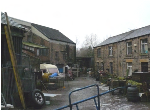
Figure 69 North Elevation of Main Block and Narrow Two-Storey Building
