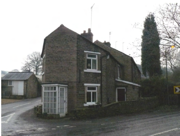
Figure 64 Toll Bar House
