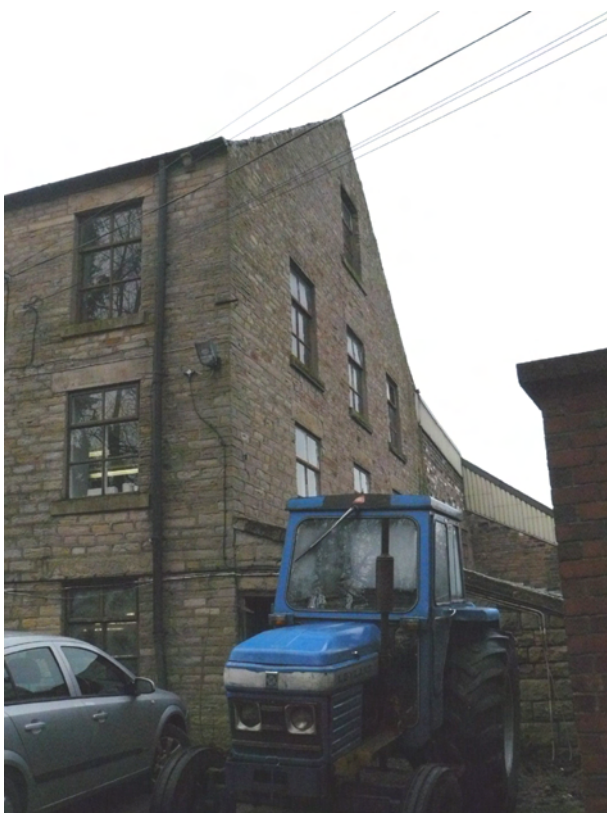
Figure 67 North Gable of Original Building
