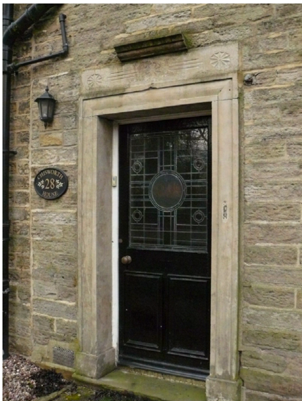
Figure 66 Door of Chisworth House
