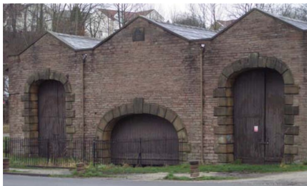
Picture 22 Front elevation of the warehouse building
