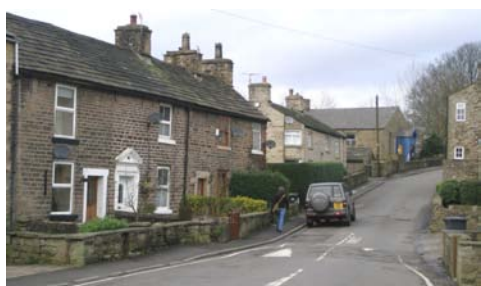
Picture 58 55 - 63 Old Road
