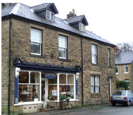
Picture 13 A well detailed and maintained traditional shopfront on George Street
