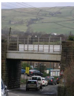
Picture 43 View from Reservoir Road with surrounding hills in the distance
