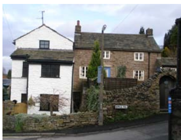
Picture 55 40 and 42 Old Road
