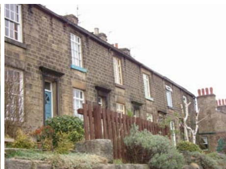
Picture 46 Terraces along Reservoir Road
