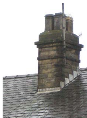
Picture 28 Chimney stack on Bingswood Avenue
