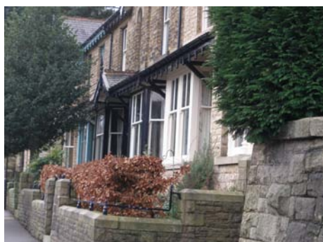
Picture 47 21 - 25 Reservoir Road - a particularly well preserved row of buildings
