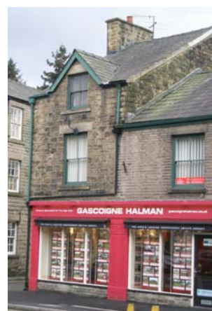
Picture 14 A well designed modern shopfront on Market Street
