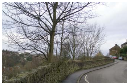
Picture 50 View along Old Road at its western edge
