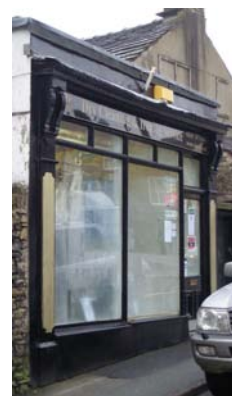
Picture 31 Shop front at 1 Bridge Street
