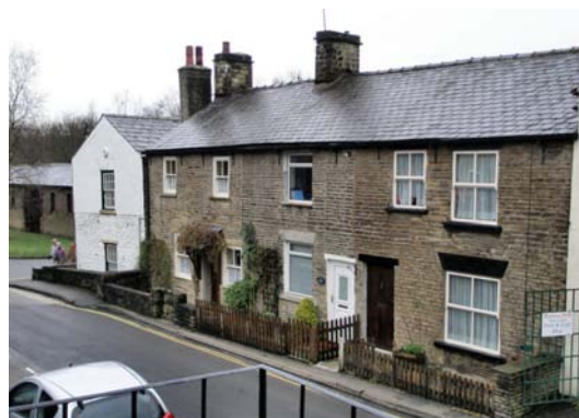
Picture 20 Cottages at the lower end of Canal Street as the area begins to open up to the canal basin
