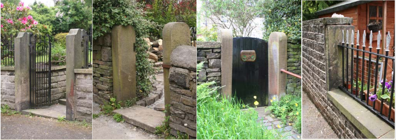
▲ Gritstone gatepiers (or stoops) and wrought iron railings in the village
