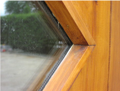
Fig 20 BS6206 'kitemarked' laminated glass fitted to this front door.
