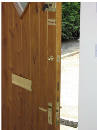
Fig 22 Door edge security showing thumb turn, five lever mortice lock rim latch and door chain.
