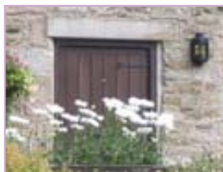
Wide door openings
