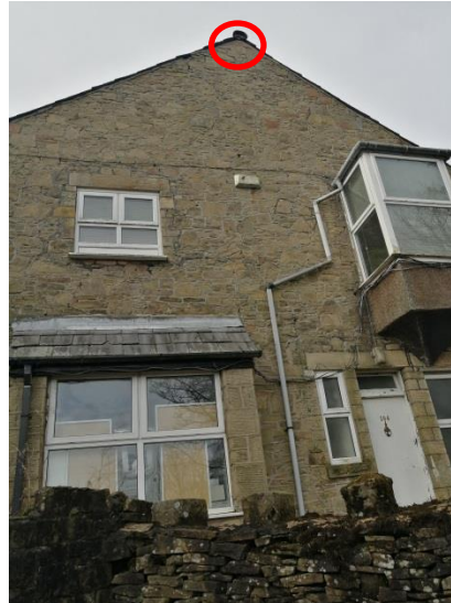
Photograph 8. The eastern elevation of the house with circled multiple features (lifted flashing, holes).
