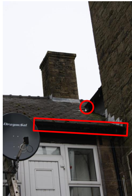
Photograph 13. Eastern elevation with some gaps to edge allowing potential access to behind wooden cladding (marked).
