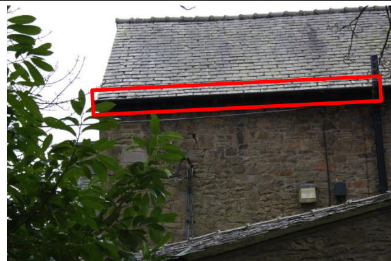
Photograph 14. Western elevation of the main building with bat potential under soffit board (marked).
