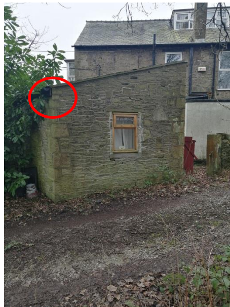
Photograph 18. Shed building with the wooden barge board (circled).
