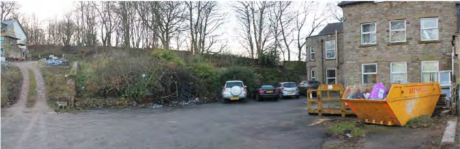
Photo 9 Main building and car park plus elevated garden area beyond the cars
