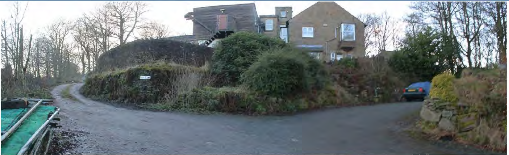
Photo 5 Looking up from the driveway to the main building showing changes in ground level
