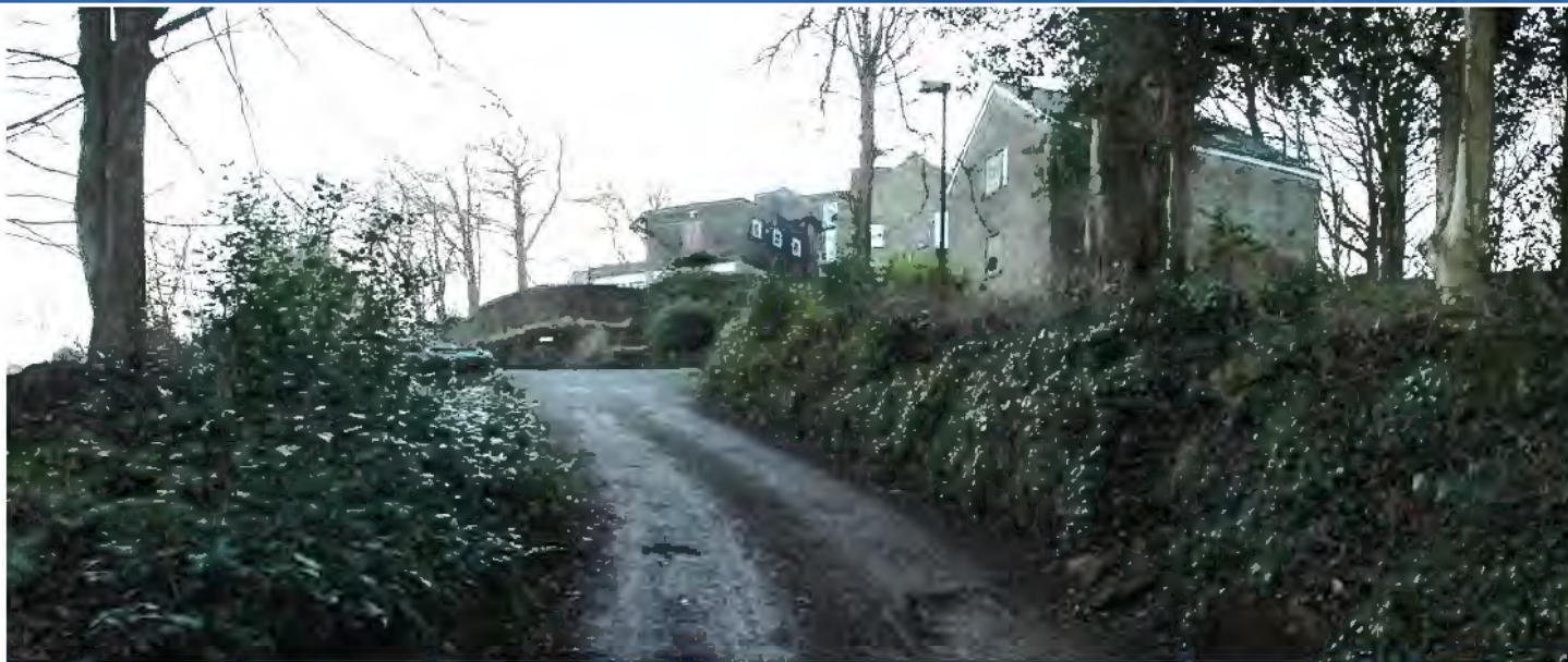
Photo 2 The site access drive looking towards the garage and the main building behind
