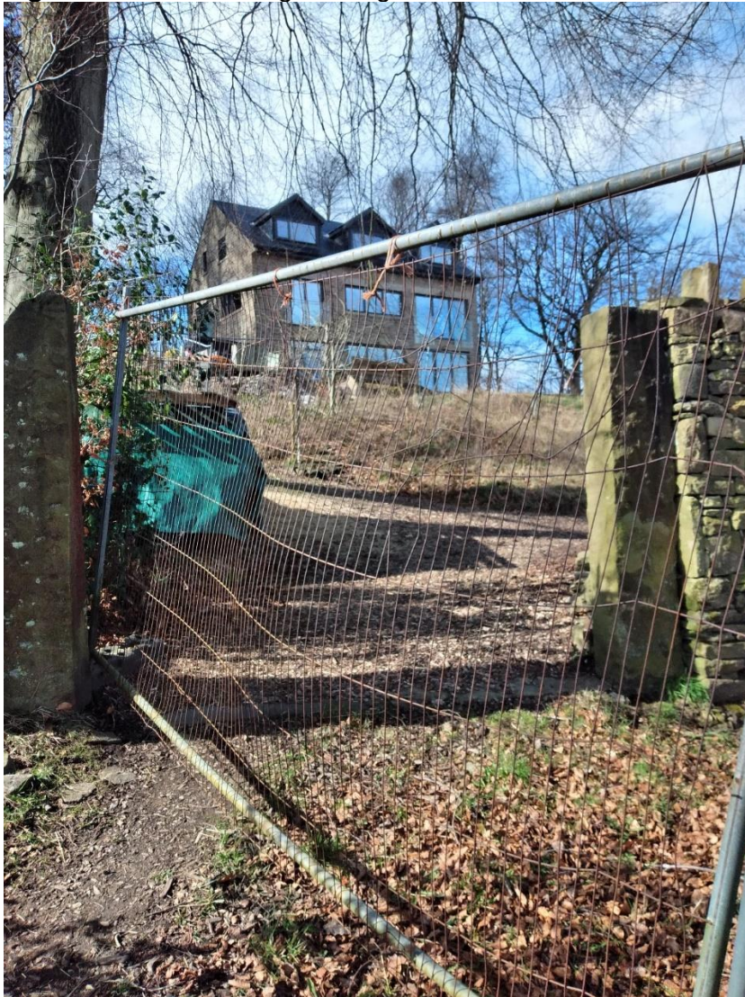
Fig 18 – View of existing building under construction as seen from the PROW, 14/03/2022
