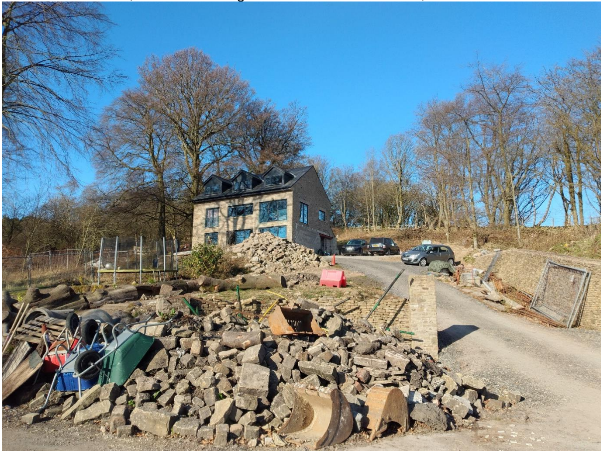
Fig 17 - The photo shows the current building in an unfinished condition with clearly exposed blockwork and lintel, there is also large amounts of rubble on site, 19/04/2021
