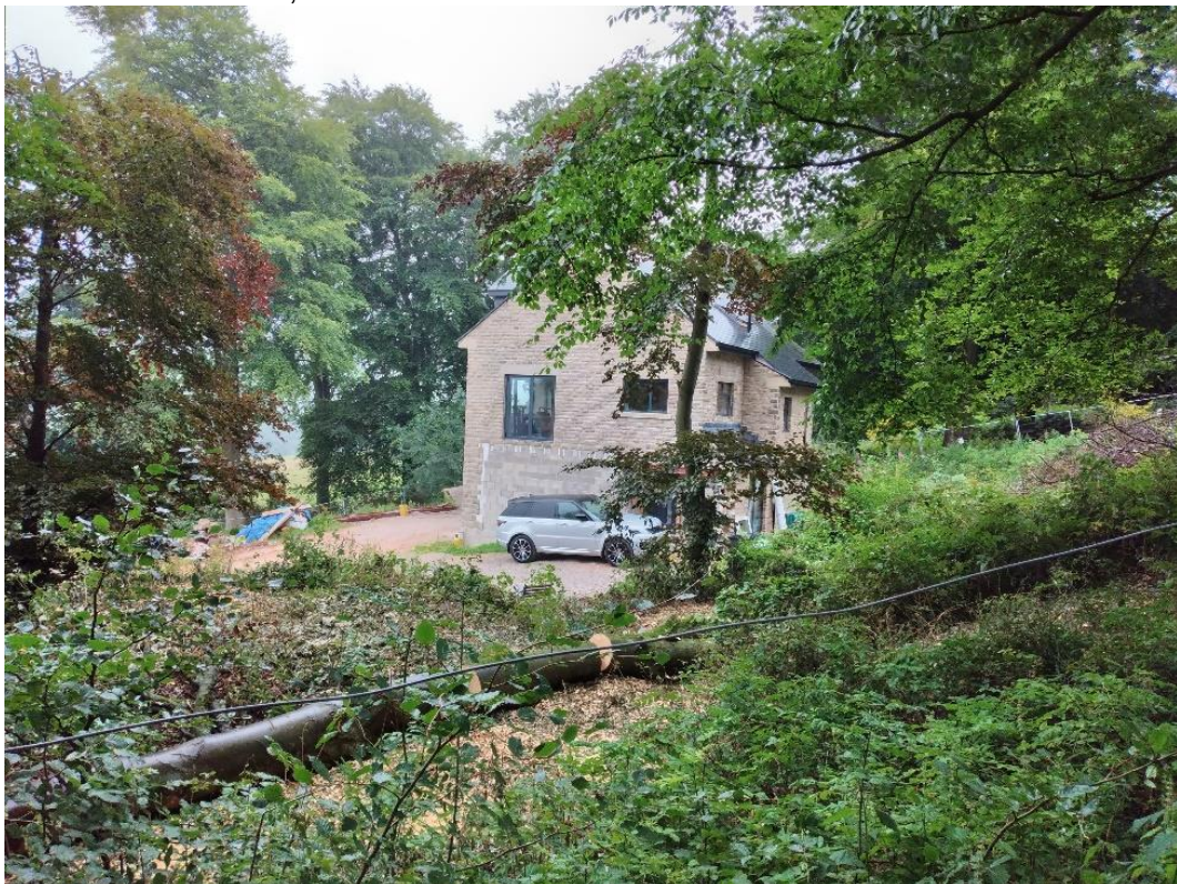
Fig 16 - The photo shows the current building in an unfinished condition with clearly exposed blockwork and lintel, 04/08/2020
