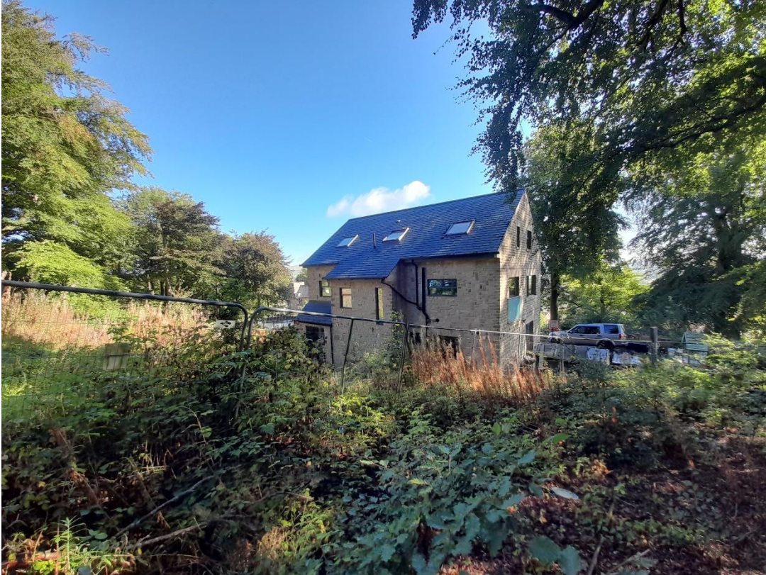
Fig 29 - The South-West corner, 23/09/2022
