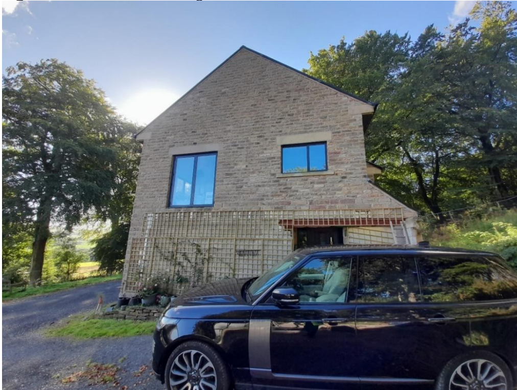
Fig 31 - North elevation facing the Edwardian house, 23/09/2022
