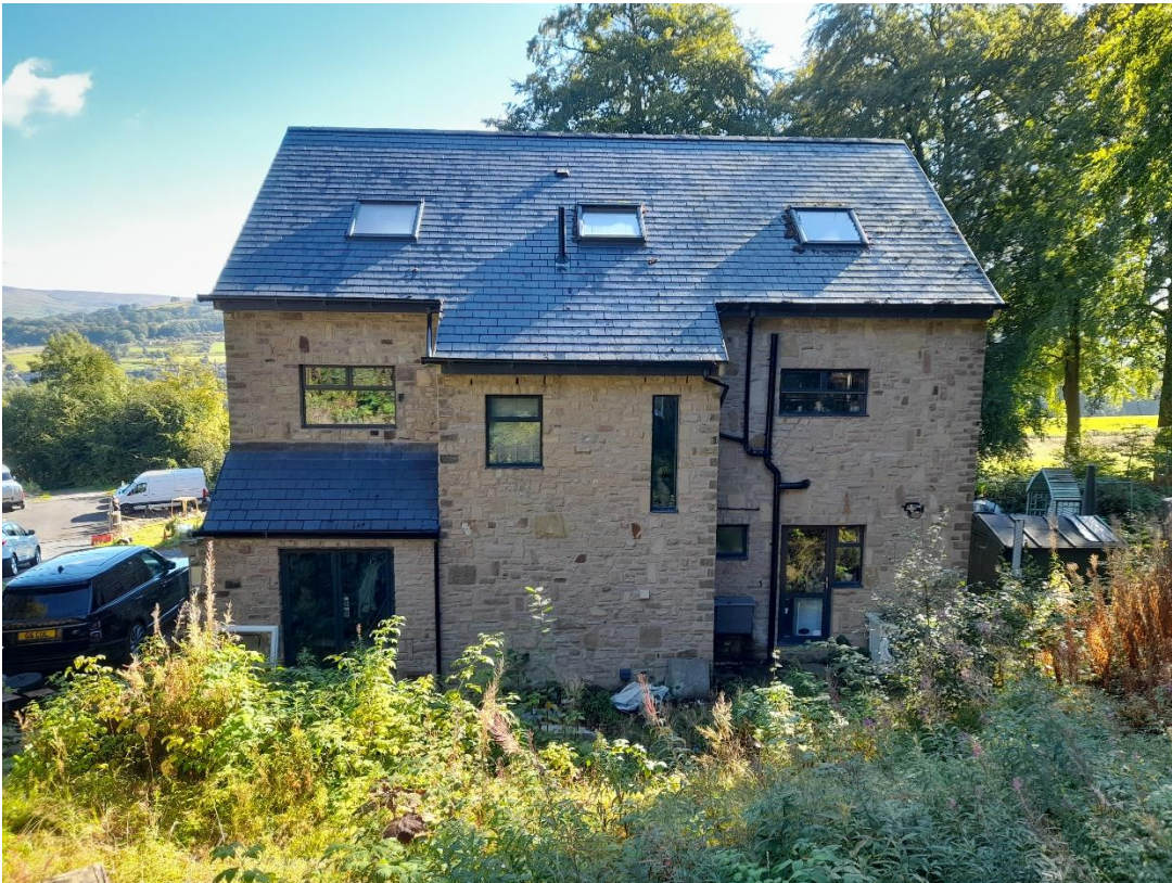
Fig 30 - West elevation (facing the rear slightly uphill towards forestry commission land), 23/09/2022
