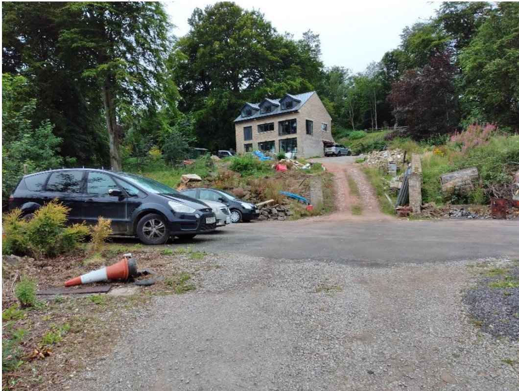
Fig 15 - The photo shows the current building in an unfinished condition with clearly exposed blockwork and lintel, 04/08/2020
