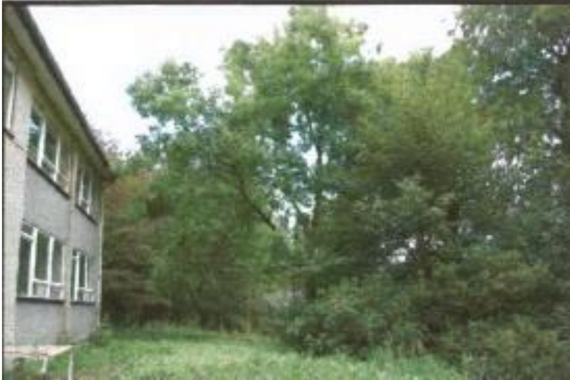
Fig 8 - Photographs of Classroom Block, from an Appraisal of Trees, September 2009
