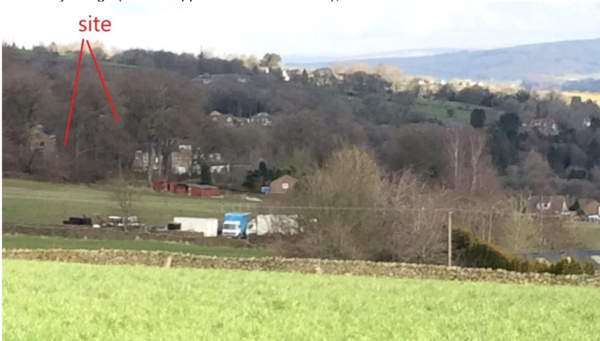
Fig 20 - View of the current building as viewed from 730m south of the site from the PROW at Whaley Bridge (the two appeal sites are labelled), 06/03/2022
