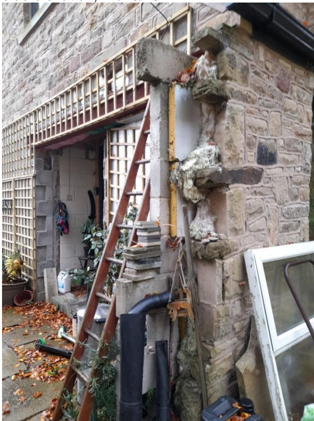
19 Section of breeze blocks positioned in a perpendicular position to the north side elevation, 27/10/2022
