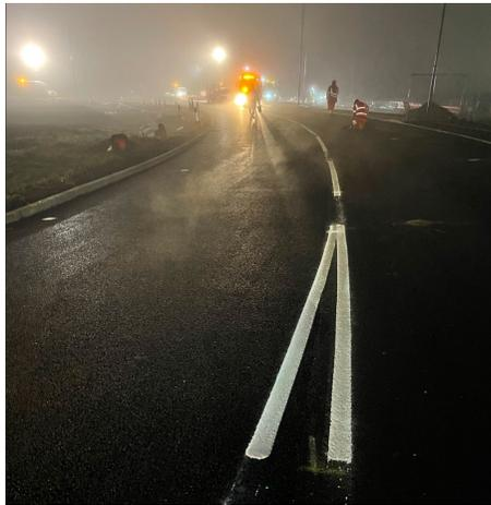
During November and December the Galliford Try site team have been able to overcome a number of challenges and complete the works as planned. The culmination of this was a week of night closures on the A6 to allow for the final layer of surfacing to the new carriageway. Thankfully this operation was completed during the favourable winter weather and before this period of colder temperatures.
