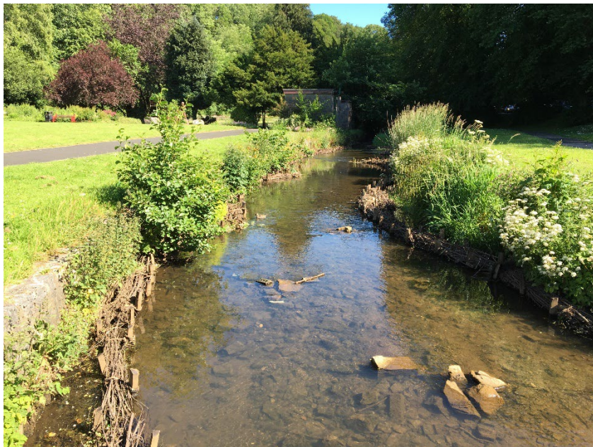
Coir roll installed in the river to divert flow and create meanders
