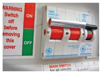
The main switch is normally the switch as shown in the photograph above and cuts off all the power to the circuit breakers / fuses.
