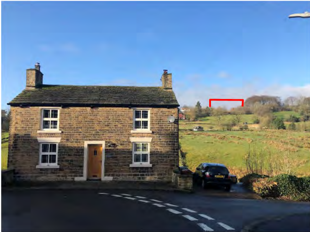
Figure A2.3: View along Blackshaw Road towards junction with Thorpe Street
