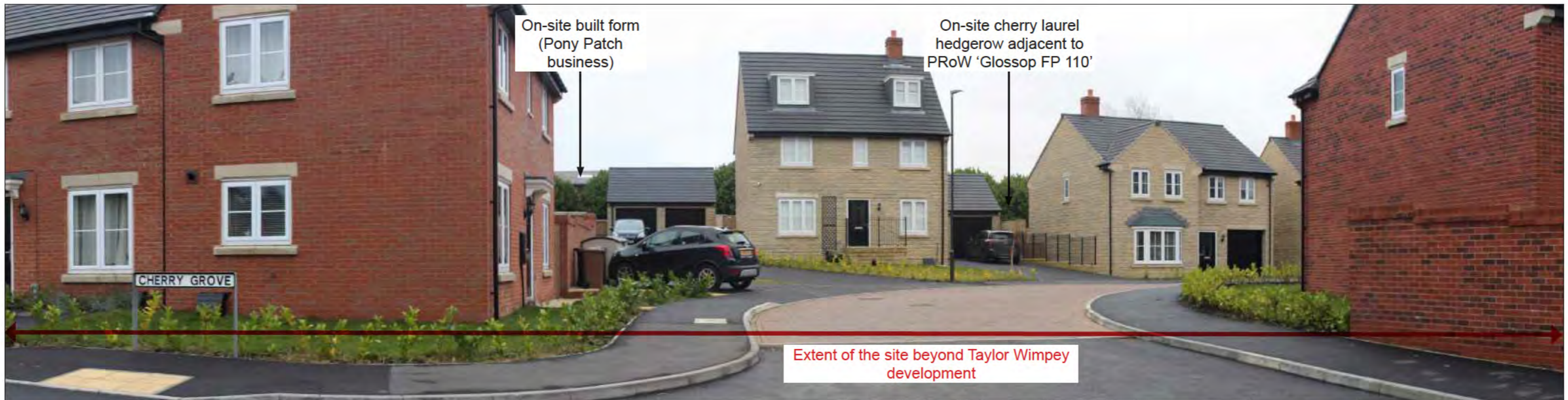
Photoviewpoint 6: Taken from the junction of Cherry Grove and Hawthorn Drive within the new Taylor Wimpey development Distance from Site: 60m Orientation: East Coordinates: SK 03421 95332
