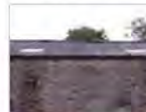
Darker roofing than walling gives weight and reduces visual impact and reflection on larger buildings
