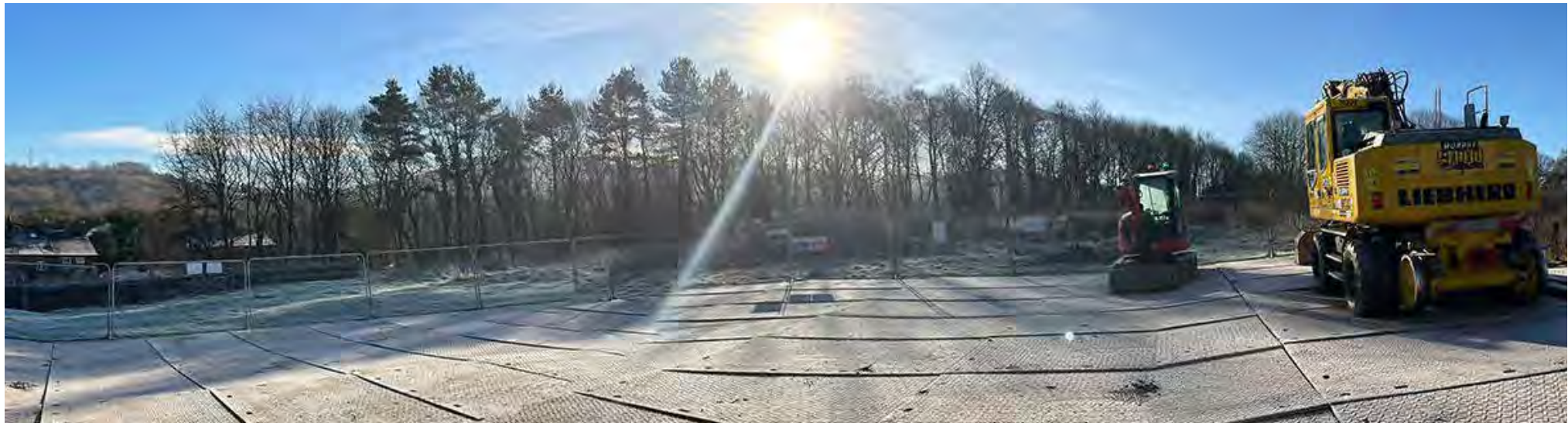
Site Photo D View from within the site looking south-east
