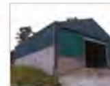
Some stone detailing helps to assimilate new development into the existing landscape setting
