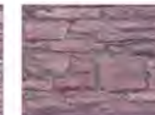
Colours should reflect those of existing, traditional gritstone buildings; warm brown tones, or deep green colours to reflect colours in the wider landscape
